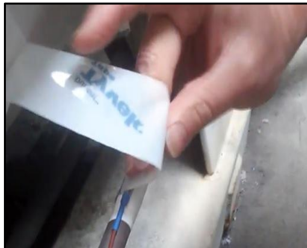
Wrap RTD sensor with Tyvek tape
