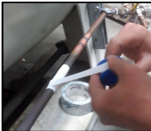
Wrap Teflon tape around 3" section of LN2 fill line
