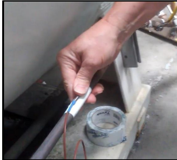
Center RTD sensor on Teflon tape
